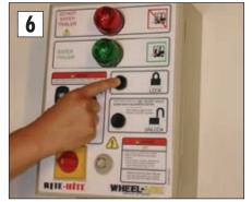
the dock attendant inside pushes the "lock" button on the control panel to activate the locking assembly.
